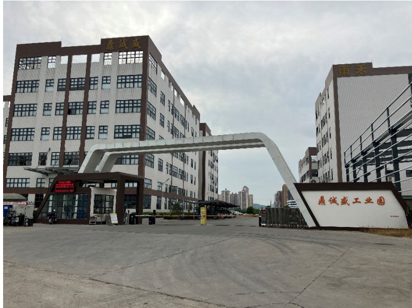
Production is primarily conducted in four production buildings
